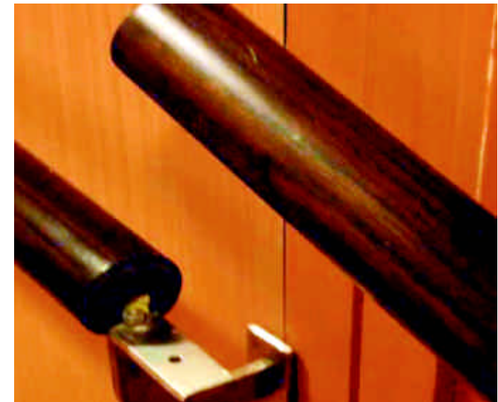
6.5.3c) A removable handrail where openings are required
