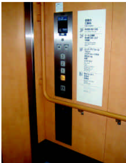
6.6.1d) Provide information of facility inside lift car
