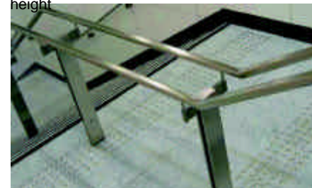
6.7.1h) Provide intermediate handrails for wide staircase that are capable of being used from both sides
