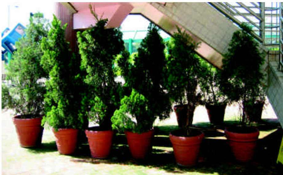
6.4.6a) Potted plants put under the stairs as a remedial method X Should be avoided in new design
