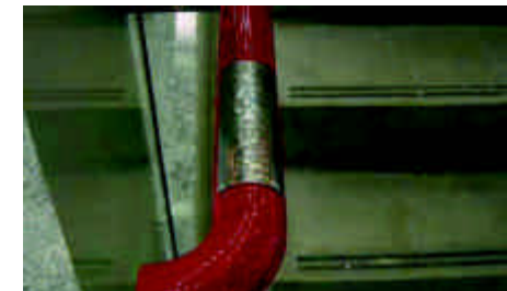
6.7.1i) End of handrail returns to the wall
