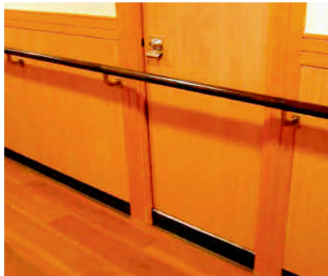
6.5.3b) Continuous handrail along corridor
