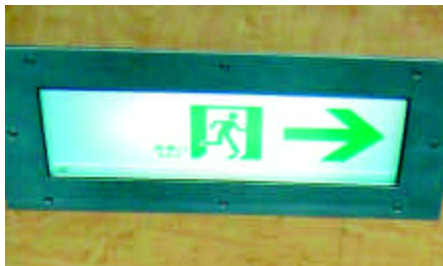
6.8.5a) Sign showing direction of exit
