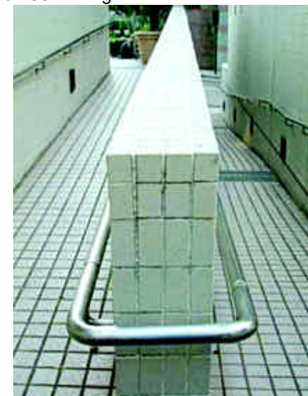
6.2.3c) Ramp with recessed light fittings and raised letters on handrails to indicate direction
