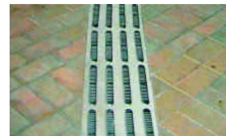
6.9.2a) Firm and slip resistant tactile surfaces
