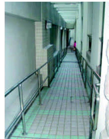
6.1.2c) Provide a ramp access to the building
