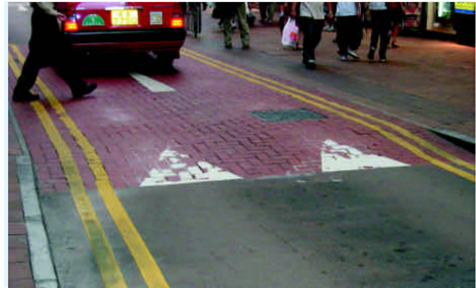
6.9.3a) Tactile warning strip at crossing
