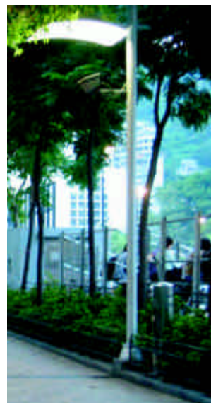
6.4.6b) Locate lighting pole outside accessible route
