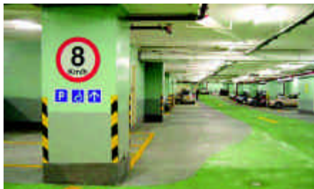
6.3.4a) Post directory sign for location of disabled car park
