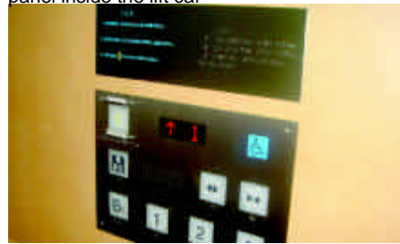
6.6.1c) Provide extended door opening control button
