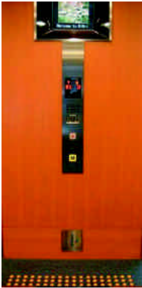
6.6.1a) Good arrangement of waiting area for lift – call button at two levels, audio and visual signaling
