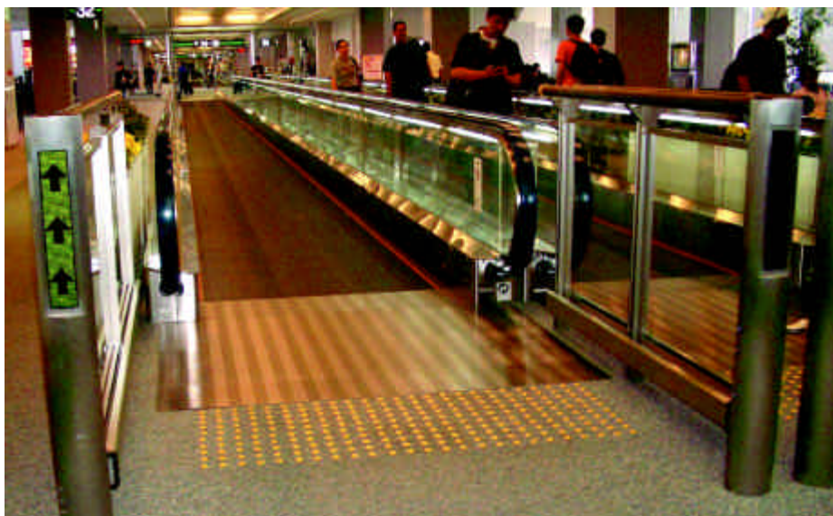
6.7.3a) Provide tactile warning strip and signage to indicate direction of travel, and align the level of the traveller with the floor level
