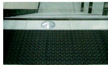
6.9.1c) Warning tile at top of staircase
