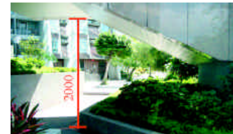
6.7.1j) Protect people from walking under part of staircase with headroom less than 2000mm with a planter design
