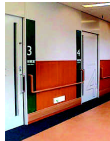
6.1.4c) Consider low level fire exit sign
