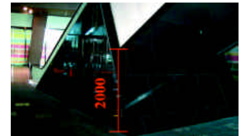
6.7.2f) Protect the underside of escalators
