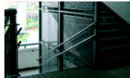
6.7.1g) Provide an additional handrail at lower height
