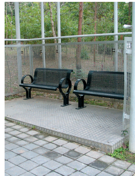
3.1.1g) Raised platform is an obstacle to wheelchair users and no warning on uneven step
