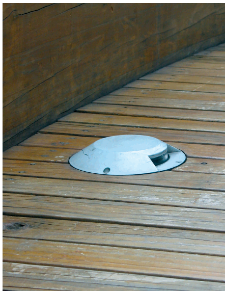
3.1.1e) Protruding fitting on ramp
