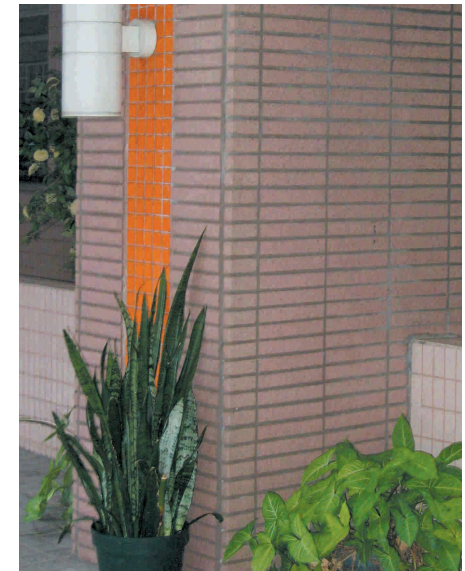
3.1.1d) Light fitting projecting on pathway with a potted plant placed below as remedial measure
