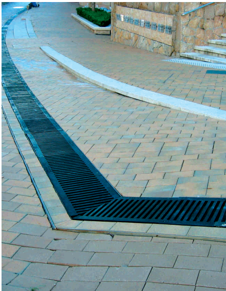
3.1.1a) Undulating pavement, uneven steps are barriers and hazardous
