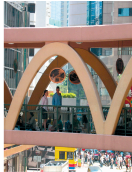
Access on elevated walkway
